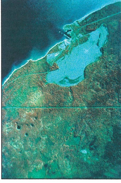
Rockport Sinkholes (aerial)
